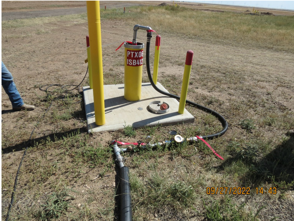
Figure 8. Offsite ISB Injection well PTX06-ISB412 with hoses for injection
