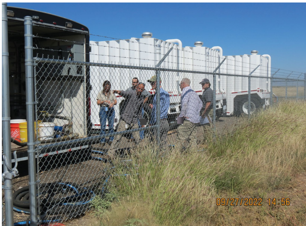
Figure 7. Offsite ISB Inspection with O&M contractor (Trihydro Corporation)
