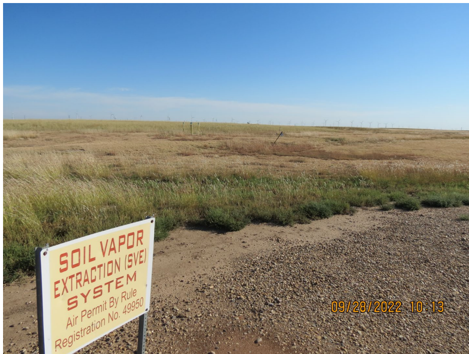
Figure 13. Burning Ground Landfill 1 Protective Cover (Beyond SVE sign)
