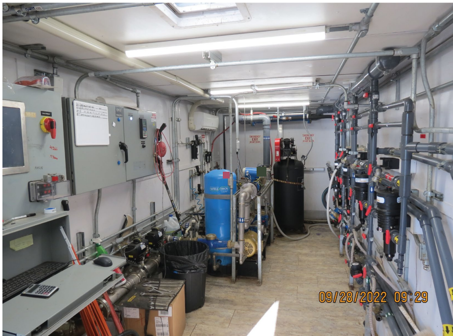
Figure 11. Zone 11 ISB mobile injection trailer
