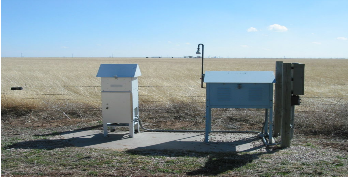
Fig. 5.3. Typical air-monitoring site.
