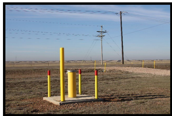
Fig. 3.20. In-situ bioremediation system well near Zone 11.
