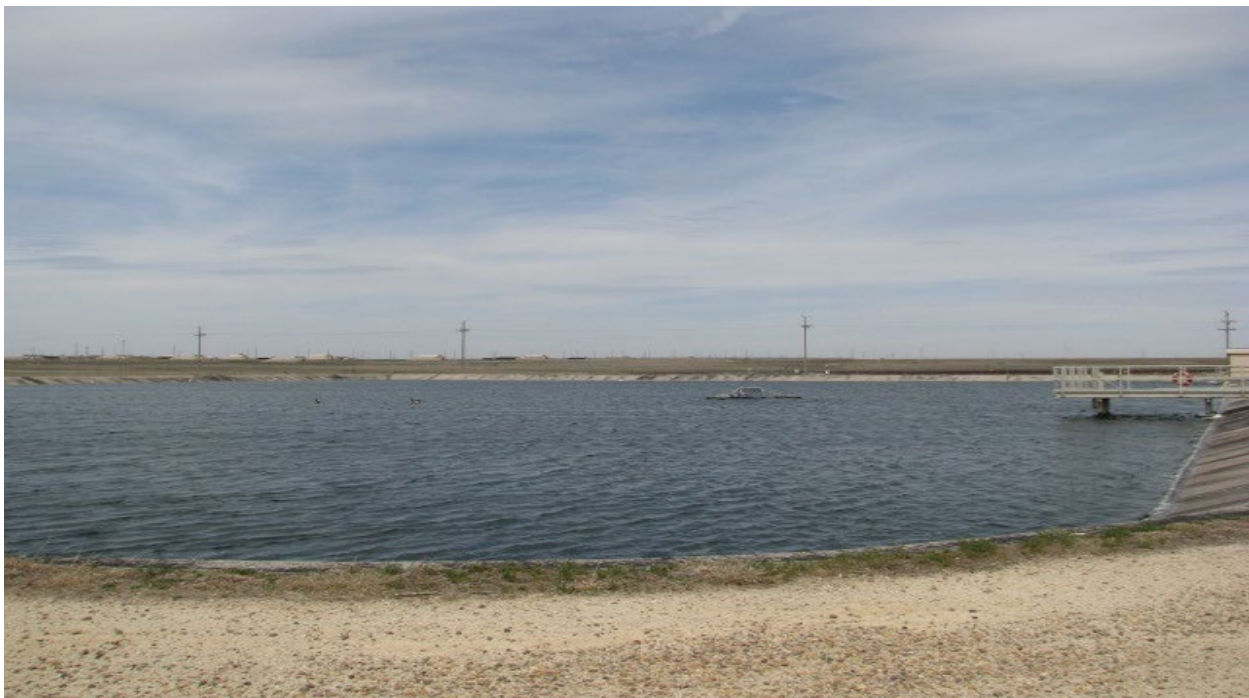
Fig. 8.4. Wastewater storage lagoon.
