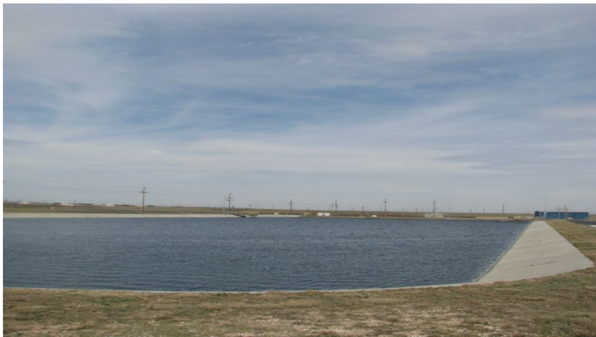
Fig. 8.2. Wastewater Treatment Facility, facultative lagoon.
