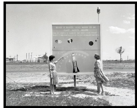
Fig. 3.11. Pantexans posing with the 8,000,000 safe hours sign.
