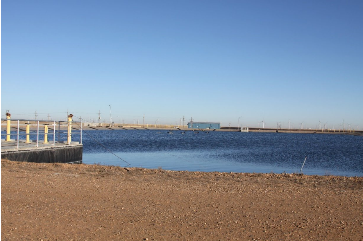
Fig. 8.3. East wastewater storage lagoon.
