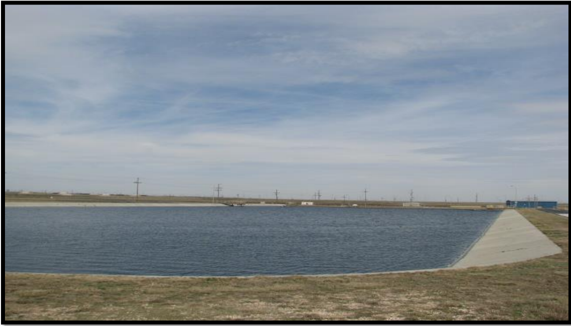
Figure 8.2 Wastewater Treatment Facility, facultative lagoon
