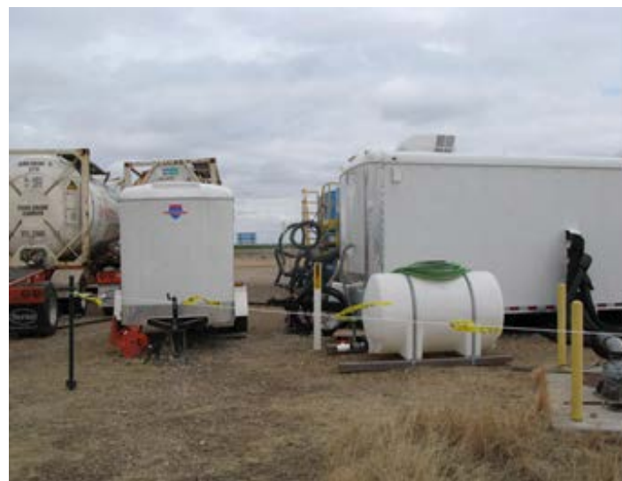
Amendment Tanks and Control Buildings at the ISBs
