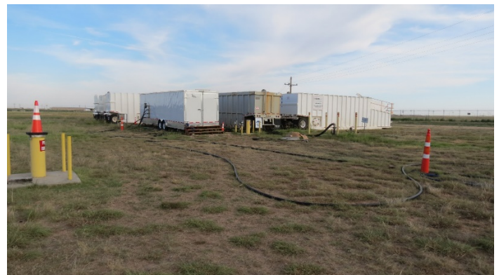
Injection Trailers at Zone 11 ISB
